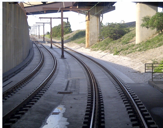
2013: Rebuilt Airport tunnel floor, drainage and tracks on Red Line
