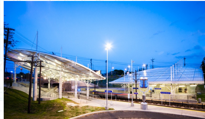
2012: Replaced Woodhill Station on the Blue & Green Lines
