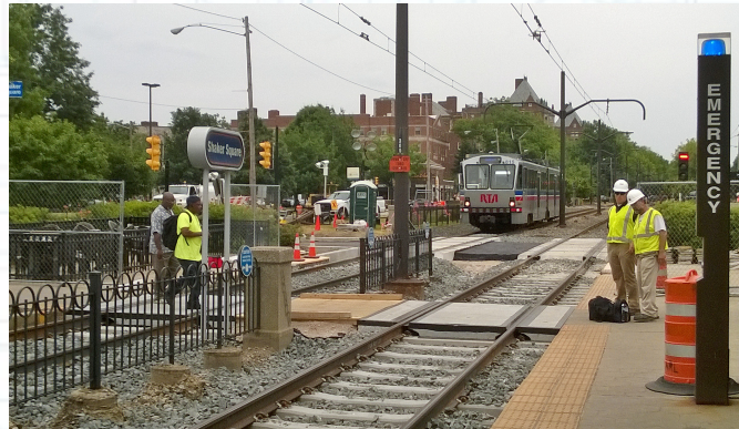
2014: replaced tracks through the Shaker Square station on the Blue & Green lines
