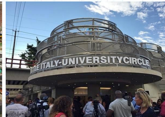
2015: built new Red Line station at Little Italy-University Circle
