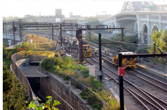
2010-2015: State-of-good-repair work to improve track and bridges system-wide
