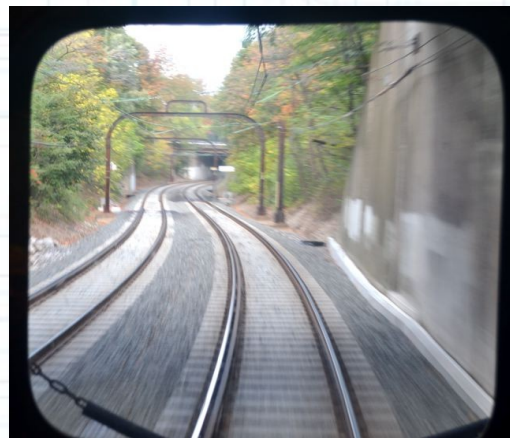
2013: Rebuilt Red Line S-Curve between West Blvd & West 117 th
