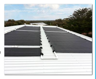
The pool itself is approx 136 sqm in area with no other form of heating, except for a solar blanket. There was no separate solar plumbing incorporated in the pool, so the solar system was plumbed via the existing filtration lines.
