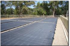
With insufficient roof space available for the installation of the entire solar equipment, the Council agreed to fence off and seal some ground space on the slope behind the filtration equipment building. Heliocol was then able to install sufficient square metres of panels to supply the solar savings for the 50 metre pool. The separate solar system for the undercover 25 metre pool was installed on the pool's own curved fibreglass roof.
