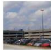
ATL International Airport N. Terminal Parking Deck
