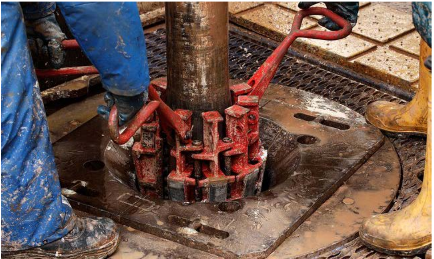
Engineers at work on the drilling platform of the Cuadrilla shale fracking facility in Preston, Lancashire. Photograph: Matthew Lloyd/Getty Images
