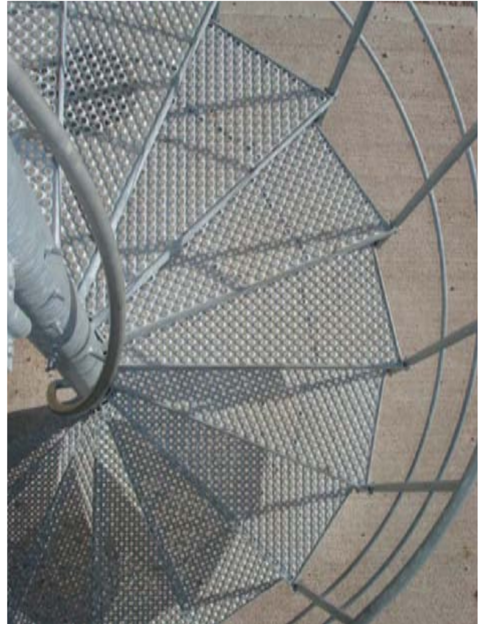
spiral with non-slip perforated steel treads
