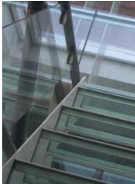
half turn commercial stair with glass treads
