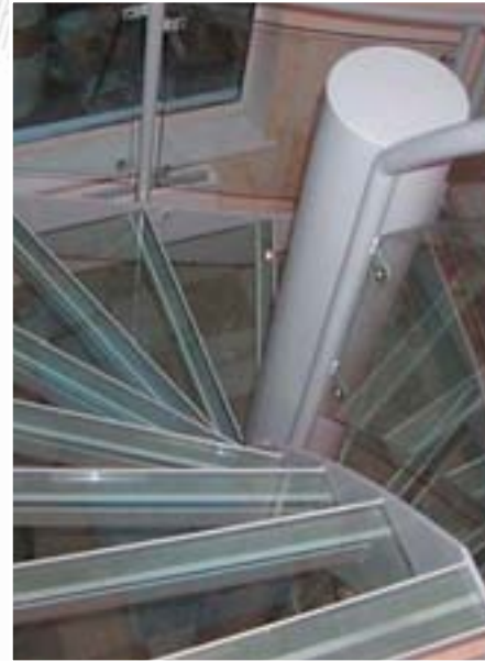
domestic half turn stair with glass treads
