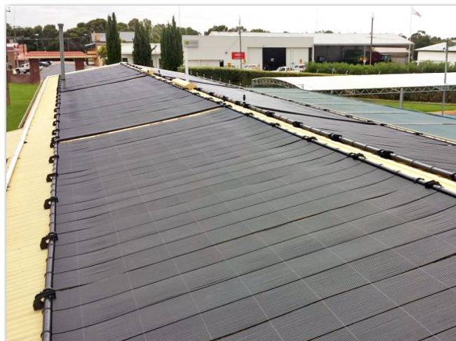
New Heliocol solar pool heating system.
