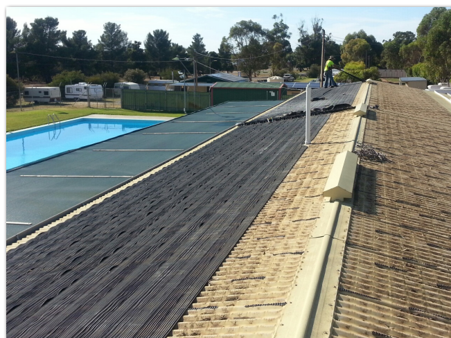
Removing old rubber strip collectors.
