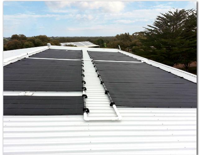
The pool itself is approx 136 sqm in area with no other form of heating, except for a solar blanket. There was no separate solar plumbing incorporated in the pool, so the solar system was plumbed via the existing filtration lines.
