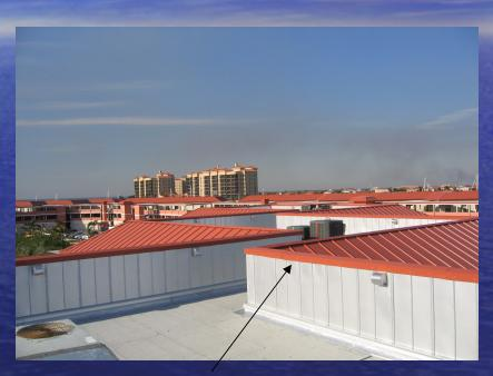
Mounts on mansard wall (not roof) just like a satellite TV dish (on the board-endorsed engineered mounting bracket) Cable to apartment via a short run paint color-matched low profile surface mount channel virtually invisible to the casual observer
