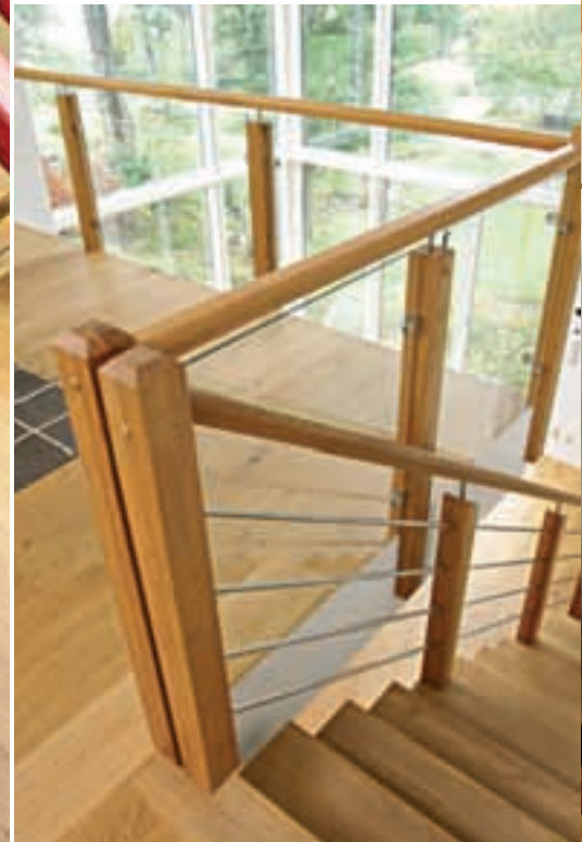
Spirit Design, Straight staircase in oiled oak, with horizontal spindles in stainless steel and laminated-glass landing balustrade
