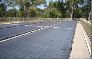
install sufficient square metres of panels to supply the solar savings for the 50 metre pool. The separate solar system for the undercover 25 metre pool was installed on the pool's own curved fibreglass roof.
