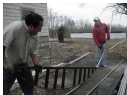
Bend and set rafter into ground post
