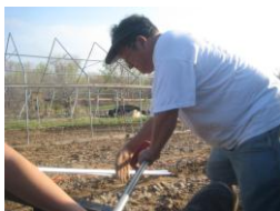
Cutting rafter into length
