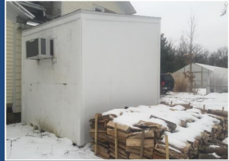
DIY Walk-in Cooler w/Air Conditioner
