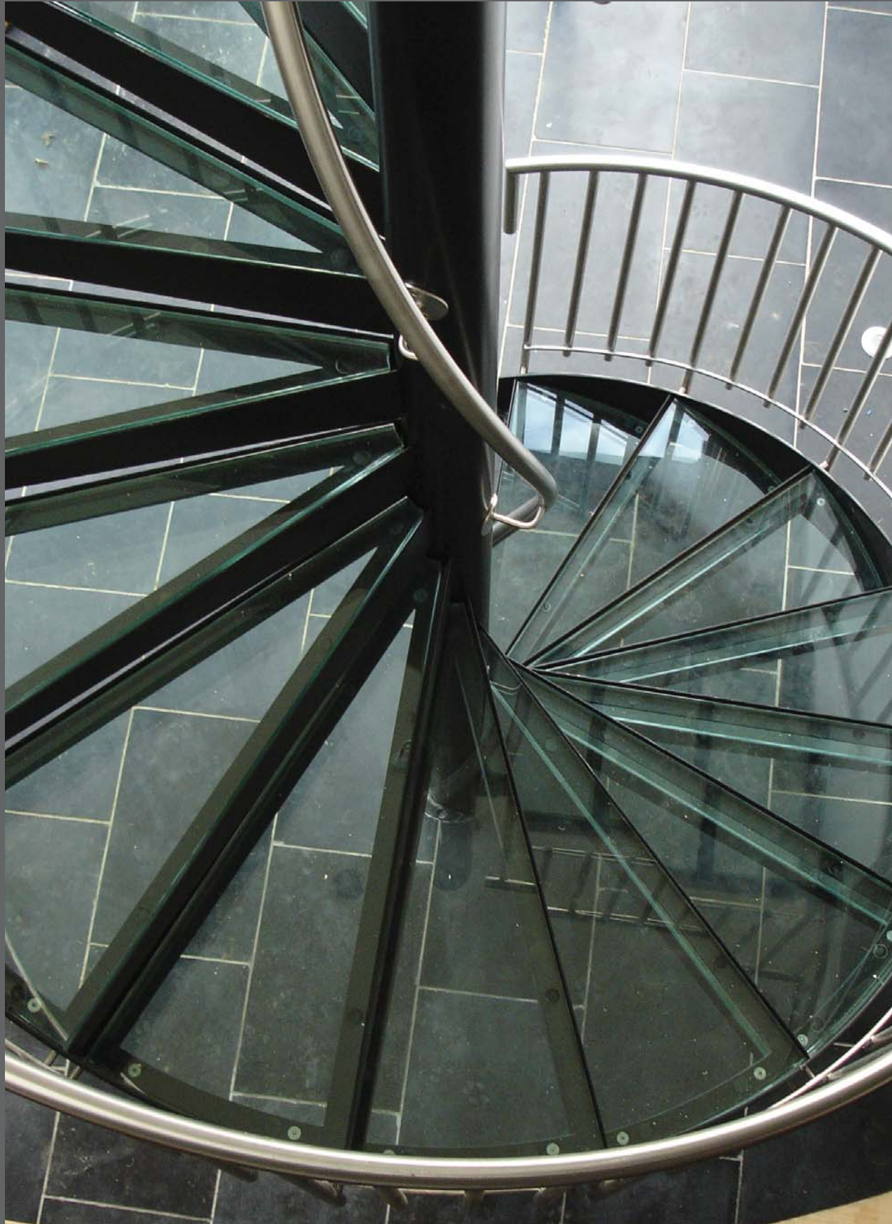
Main picture: Spiral with laminated glass treads in steel frame. Steel stringer and stainless spindles.
