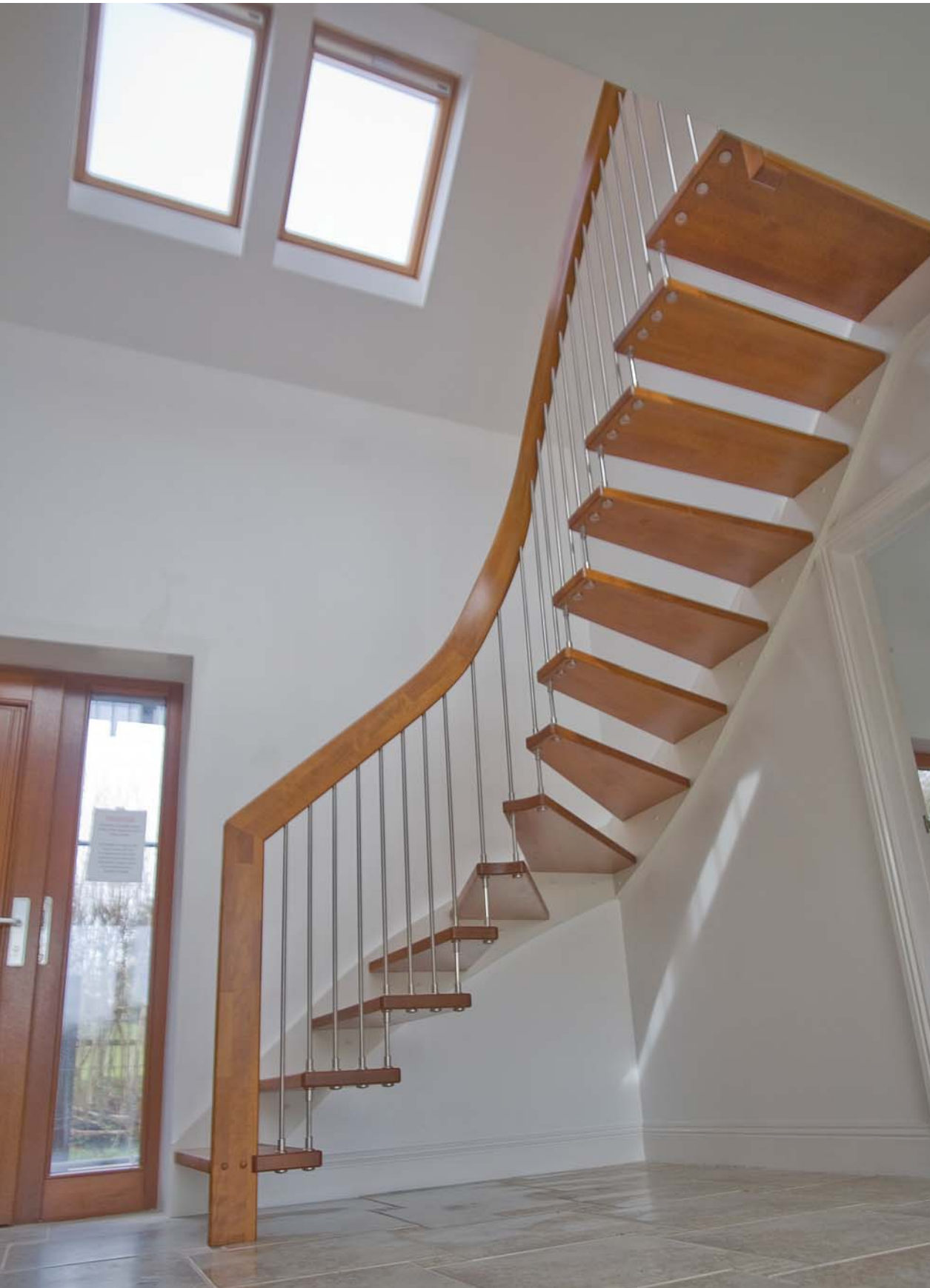
Main picture: Quarter turn WF Staircase with beech treads. White wall stringer and curved internal handrail.
