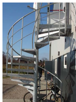
Bottom right: Spiral fire escape for a factory. Horizontal balustrade, fully galvanised.
