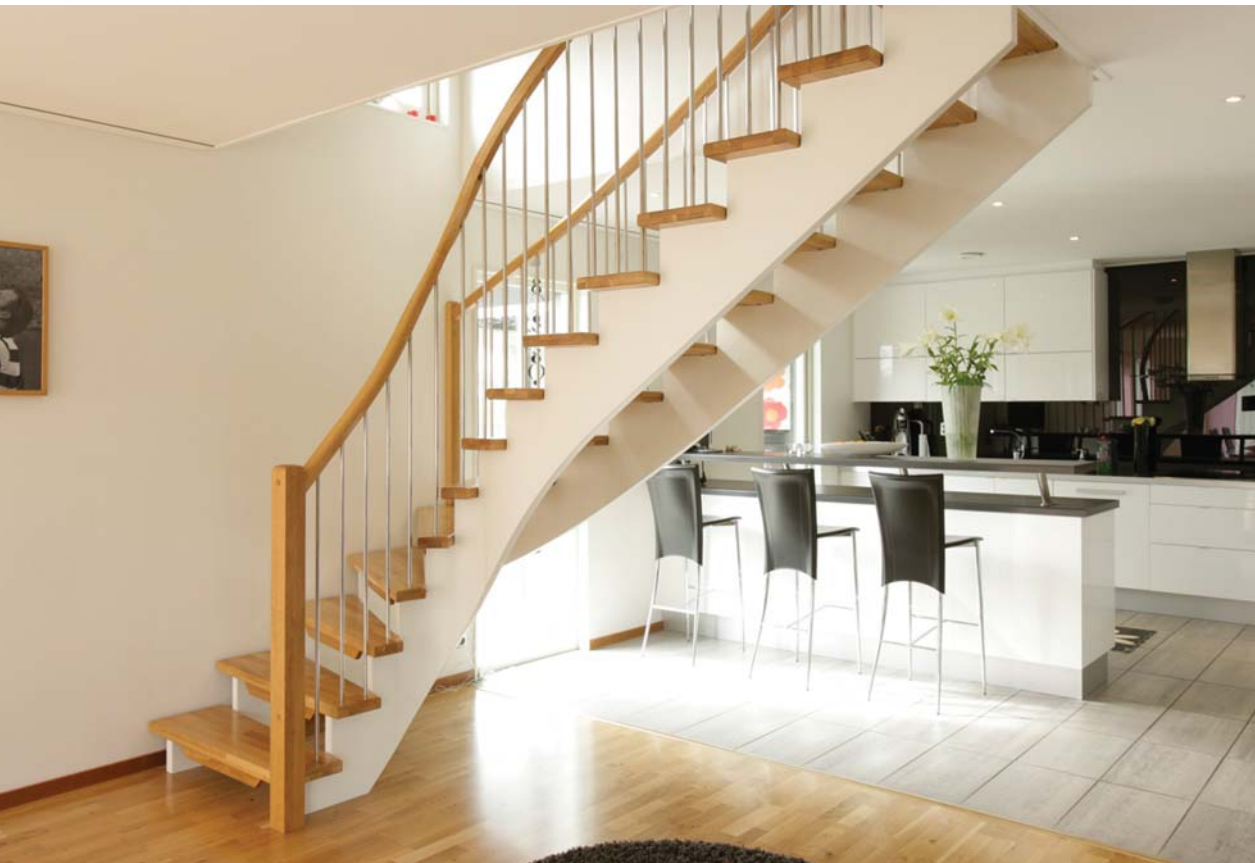
Main picture bottom: Quarter turn stepped stair with oak treads, white stringers and curved handrail.
