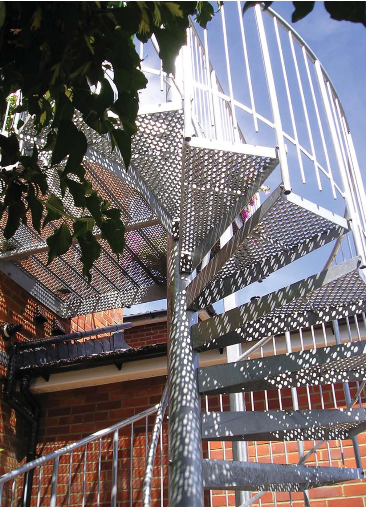
Main picture: Domestic fire escape and balcony with non slip perforated treads and deck.
