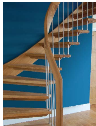
Bottom right: Quarter turn WF Staircase with oak treads, stringer and handrail. Curved internal handrail and stainless spindles.
