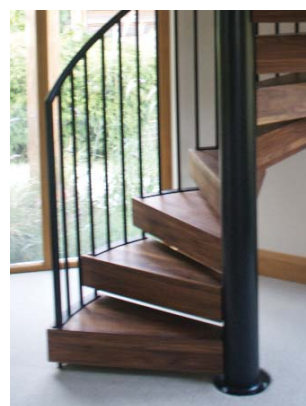
Bottom right: Spiral with boxed style walnut treads and vertical steel spindles.
