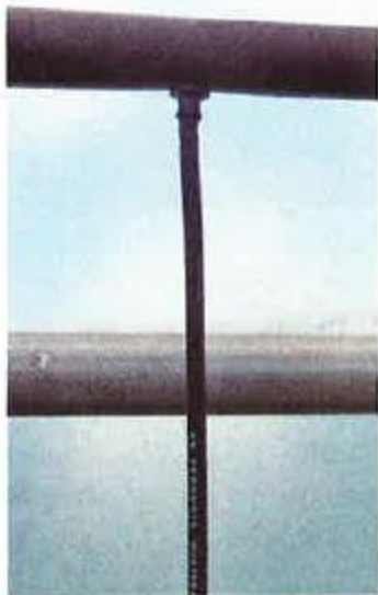
Figure 6. 1/4-inch dropline inserted into spray supply line
